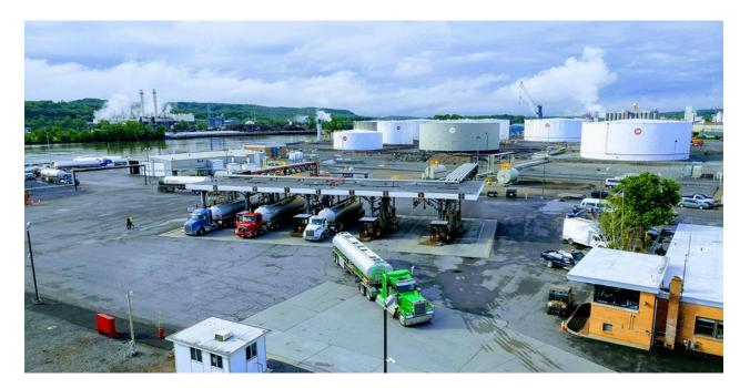
Global's Albany Terminal is a barge, rail, and truck supplied terminal serving New York's Hudson Valley through its seven bay truck rack. The terminal is located on the Hudson River and the Canadian Pacific rail line.
