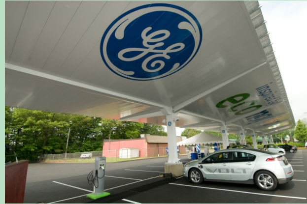
Figure 10: General Electric's Solar Carport, installed in Plainview, Connecticut (Source: GE, courtesy of C|Net).
