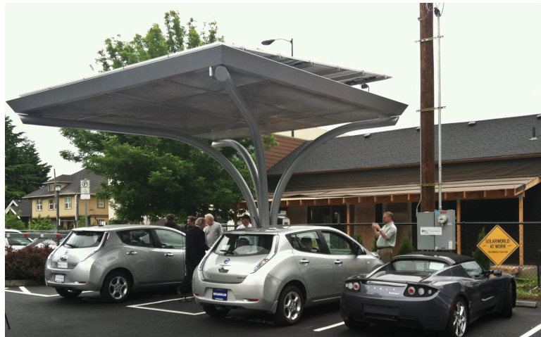
Figure 13: Solar canopy with EVSE at light rail station in Portland, Oregon (Source: Portland Development Corporation).
