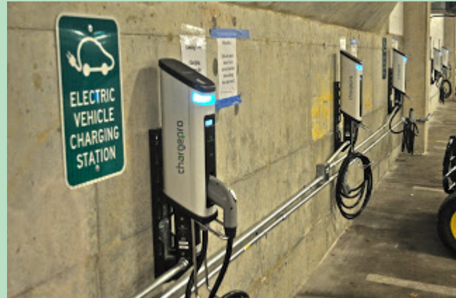
Figure 11: Wall-mounted Level 2 EVSE in JHU’s South Garage (Source: SemaConnect)
